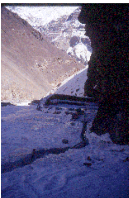
Intake kuhl to the reservoir
